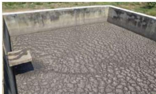
Sludge Drying Bed
