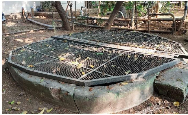
Open Well for rainwater storage
