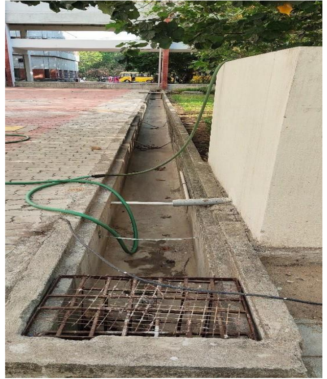
Paved Concrete Trench
